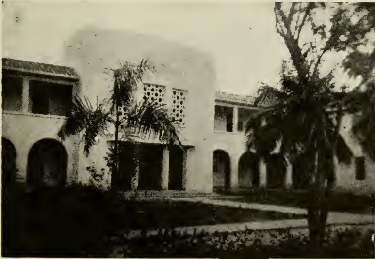
New building at George O. Robinson School, Santurce, Puerto Rico
